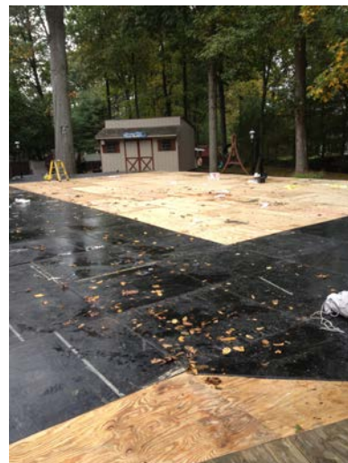
Bil-Jax staging setup and leveled to match up flush with the I beams
