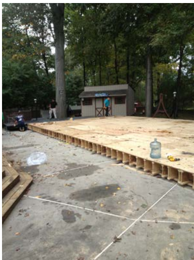
Wooden I Beams are secured to a layer of plywood for the highest level of stability over the pool area
