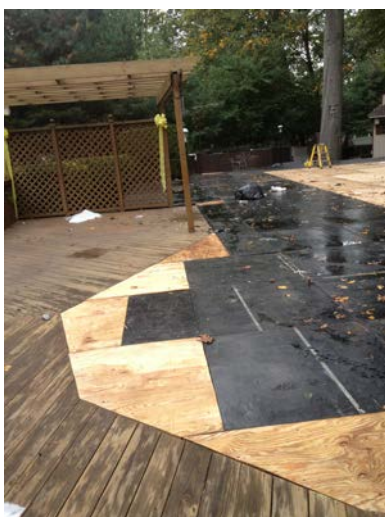
...But not for Party Line! We cut plywood and I Beams to meet the Deck and Bil-Jax evenly.
